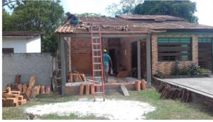
Progress on the house in Sao Luis.
